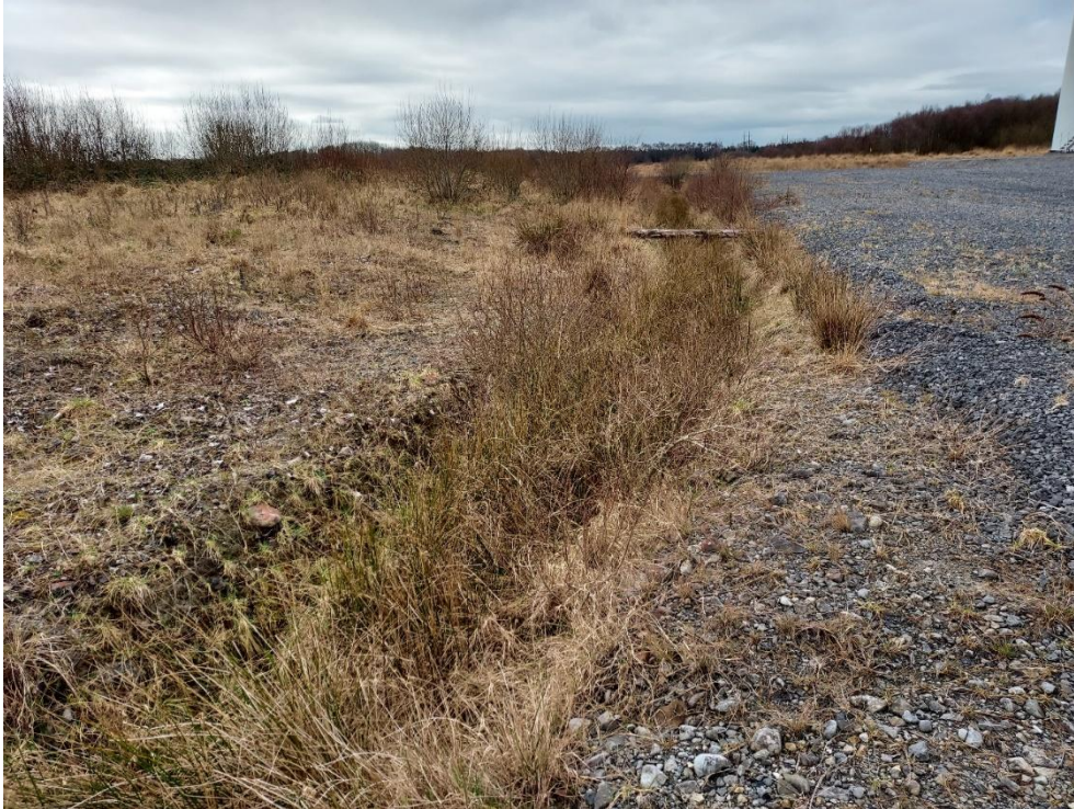
Figure 2-2 Vegetated swale
